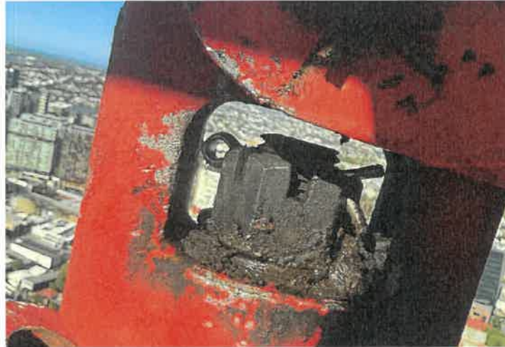
Figure 3 – Photograph showing new split pin installed through castellated nut
