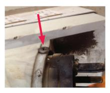
The electrical supply cable to a static boom pump must be adequately supported, to eliminate unnecessary strain on the cable and plug/socket. This can be addressed through fitting a lug
