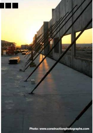
Because braces are part of a 'propriety system', grabbing a bolt on site to fill in for the correct pin is just not on.
