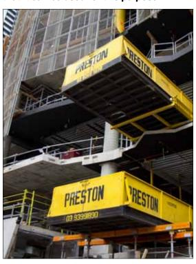
The Builder MUST also obtain INDEPENDENT engineering advice and approval for the platform to be used as a Structural Working Platform. The engineer's report must take into account all necessary LIVE and DEAD loads, and ensure that all intended loads are safely distributed.
