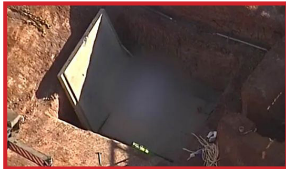
Inadequate bracing on the Eagle Farm Site resulting in double fatality
