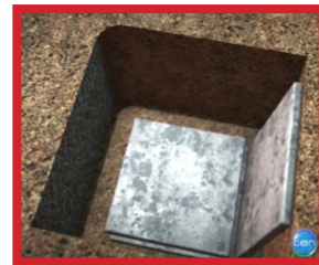
Inadequate bracing on the Eagle Farm Site resulting in double fatality
